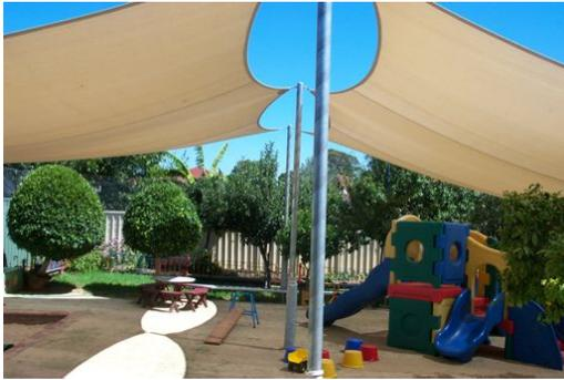
This first set of sails fails the design test. Look at the central area, the area where the shade is most important and you can see a big gap and sunlight getting through. This job has been done as two sails. It is poor design because of the light it lets in and it would have been more expensive to do it as two sails instead of a single sail.
